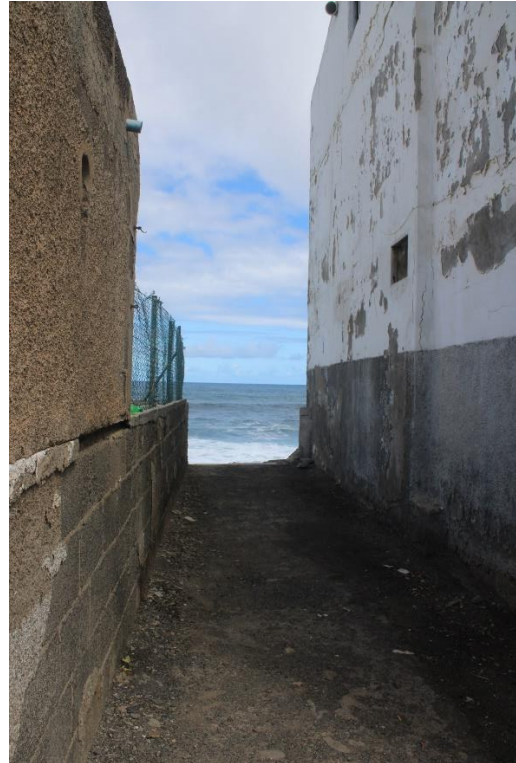
Figure 13. Acces next to pumping station
