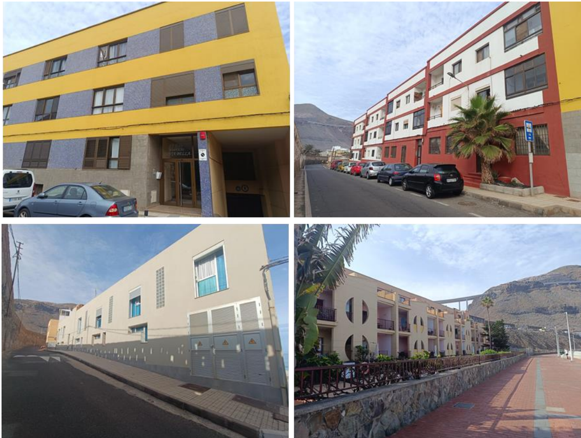
Figure 8. Photographs of the main multifamily buildings
