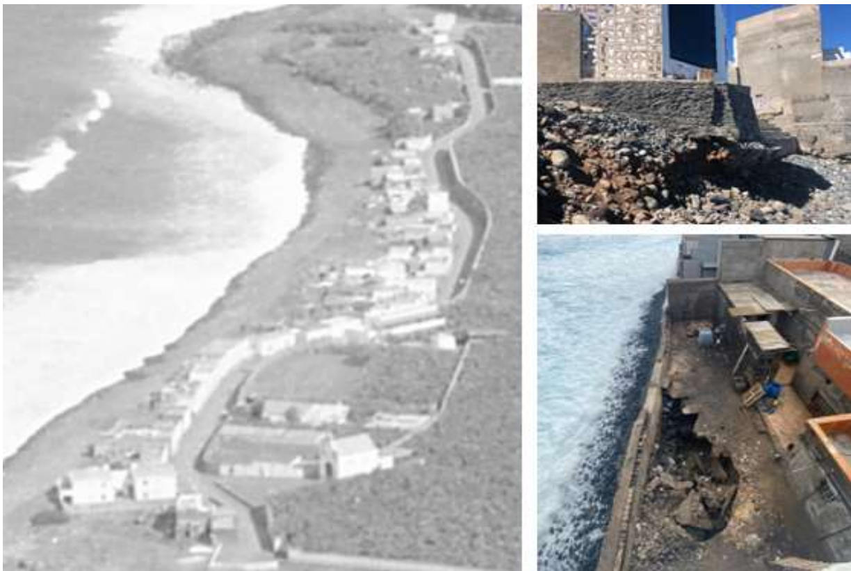
Figure 3. State of the coastline circa 1980 and current state of the buildings
